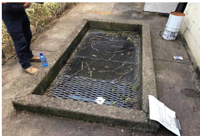
Photo 2 Existing Oil/Grease Trap
